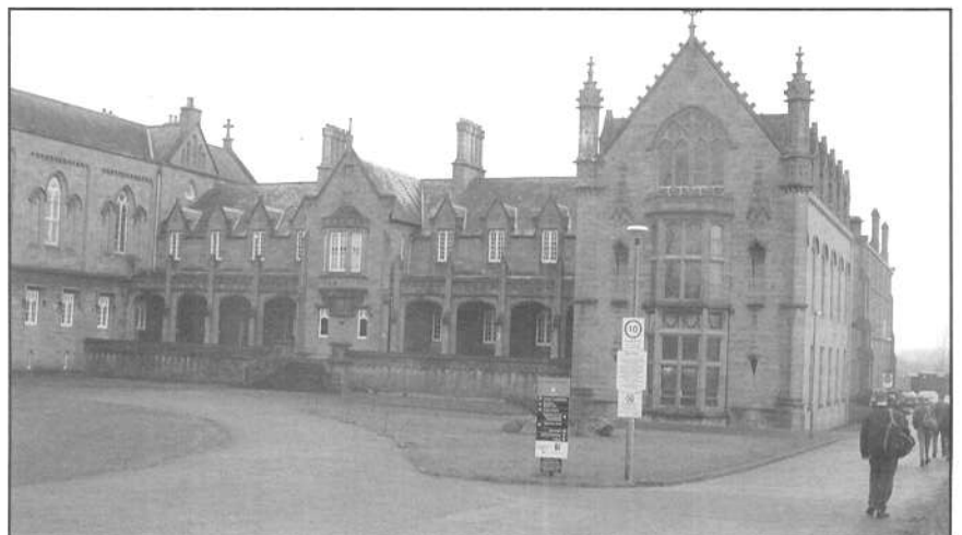
The 'Moran Wing' and the steps of the east wing were added, and both terraces were faced, in 1876-77
