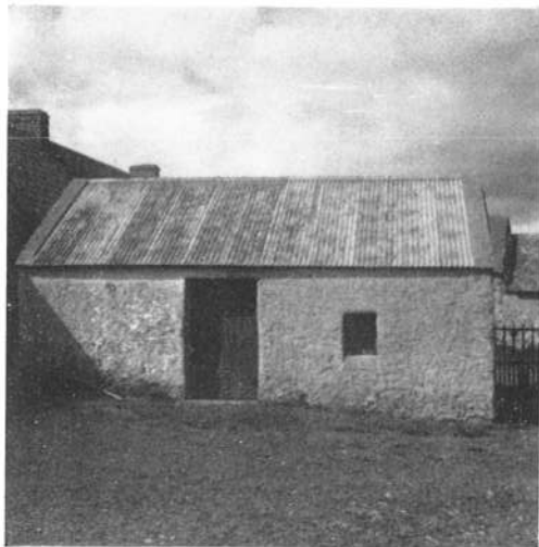
Hedge schoolhouse at Ballylinnen, Castlecomer: in use c. 1800-1812. Thatch roof replaced by corrugated iron; size 22' x 16' x 5½' externally; no fireplace; one unglazed window. Round 4' diameter stone flag mounted on masonry used as table by 20 pupils and one teacher Matt Quigley.
