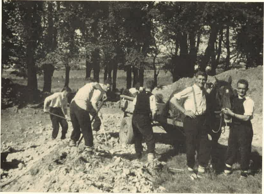
PREPARING BASKETBALL COURT
