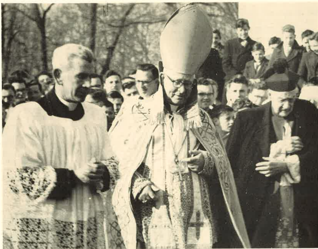
Digging first sod of Collier Wing, February 1956—BISHOP COLLIER with CANON LOUGHRY and the late DEAN CAVANAGH
